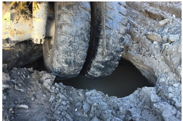
FIGURE 2: Ground collapse under wheels of loaded dump truck
