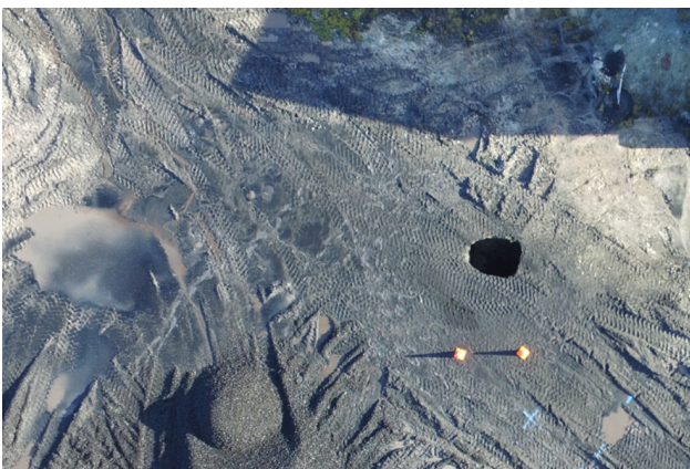
FIGURE 1: Historic underground void visible on ground surface
