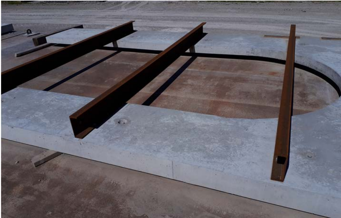
Figure 4: Strongbacks supporting a large precast concrete element
