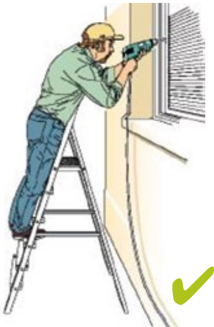
Figure 30: Correct – steps facing work activity.
