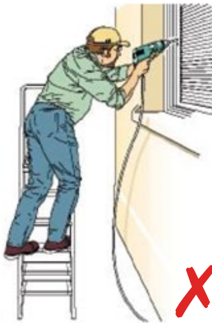
Figure 31: Incorrect – steps are side-on to work activity.
