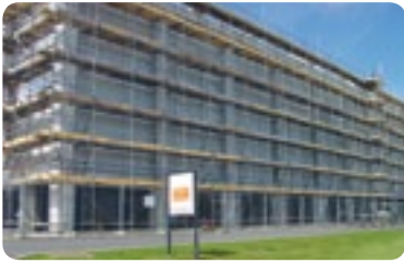
Figure 5: Scaffolding on a multi-storey building.
