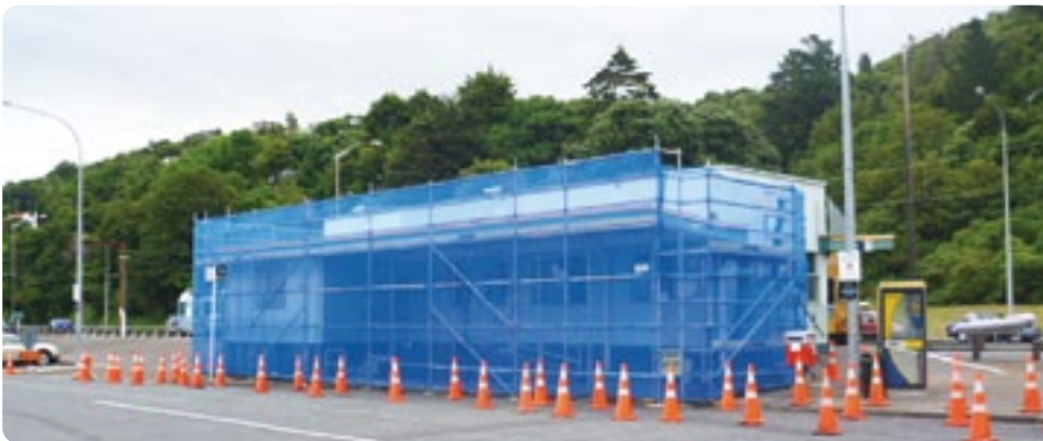
Figure 3: Covered scaffolding on a single storey building.
