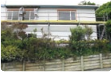
Figure 4: Scaffolding on a residential building.
