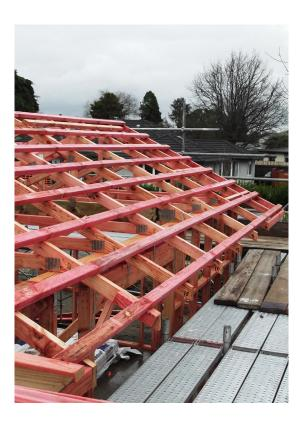
Where Inspectors find builders are relying on ceiling battens as a method of fall protection a **Prohibition Notice** will be issued requiring the builder to use a safer method of working such as temporary work platforms, safety mesh and soft landing systems.
